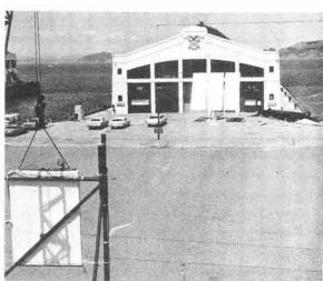
SUN DAY in SAN FRANCISCO—At Fort Mason Park on the waterfront, Dick Houser (8451) describes operation of heliostats supplied by SLL for the occasion. With Bay in background, the heliostat redirected the sun's rays to a flat-plate collector (foreground) and turned water into steam. Heliostat is Martin-Marietta design.
